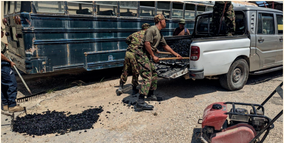
Community support missions. Road repair. Photo: official Facebook account of the Belize Defence Force.
