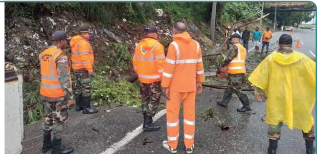
Prevention and assistance during the Franklin storm, activation of the Lightning Plan. Photo: Ministry of Defence.
